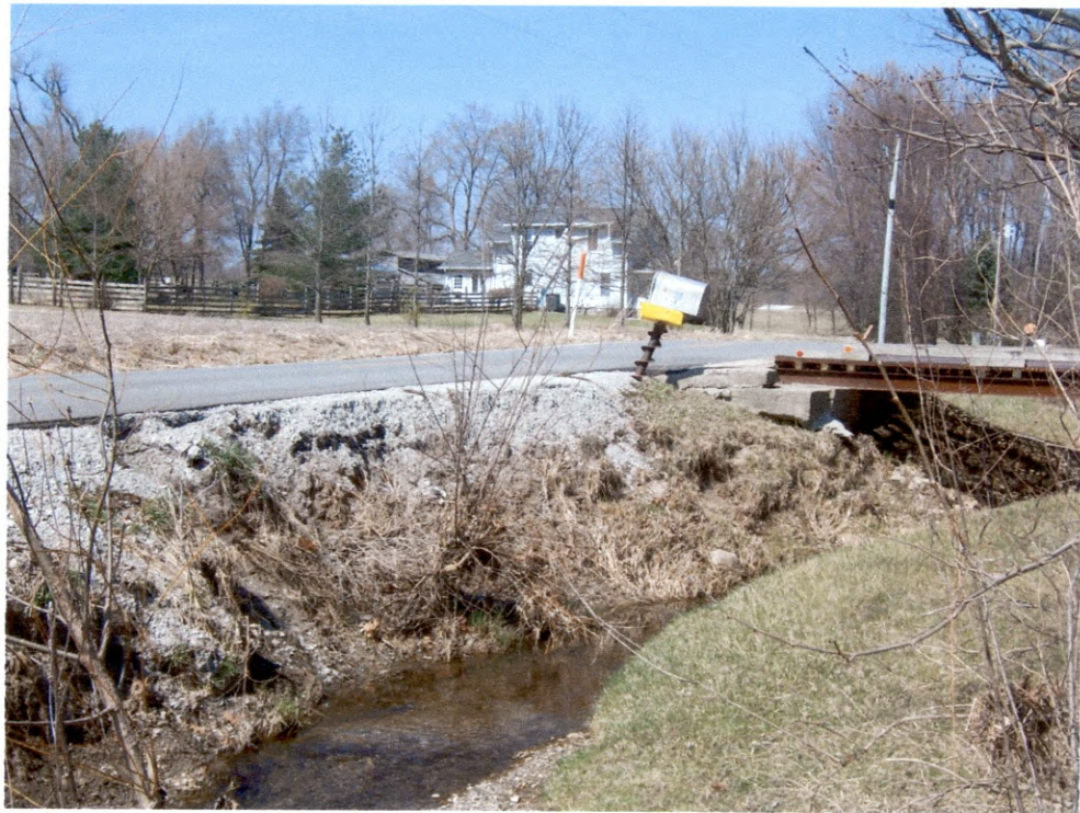
March, 2009. View from the opposite (home side) of the creek facing the road and the erosion.
