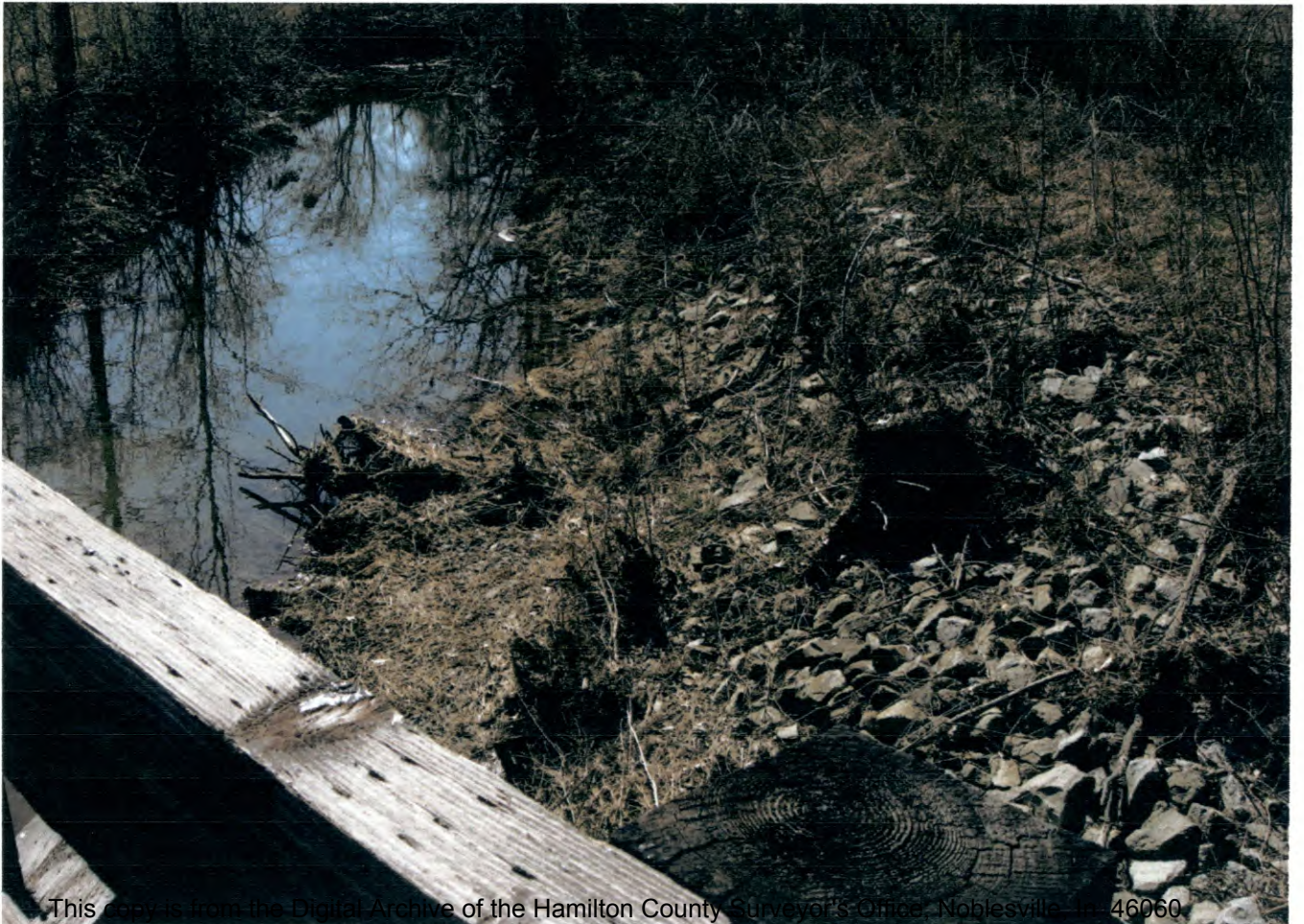
Other side of road (same bridge) riprap - County built bridge ≈ 1995
