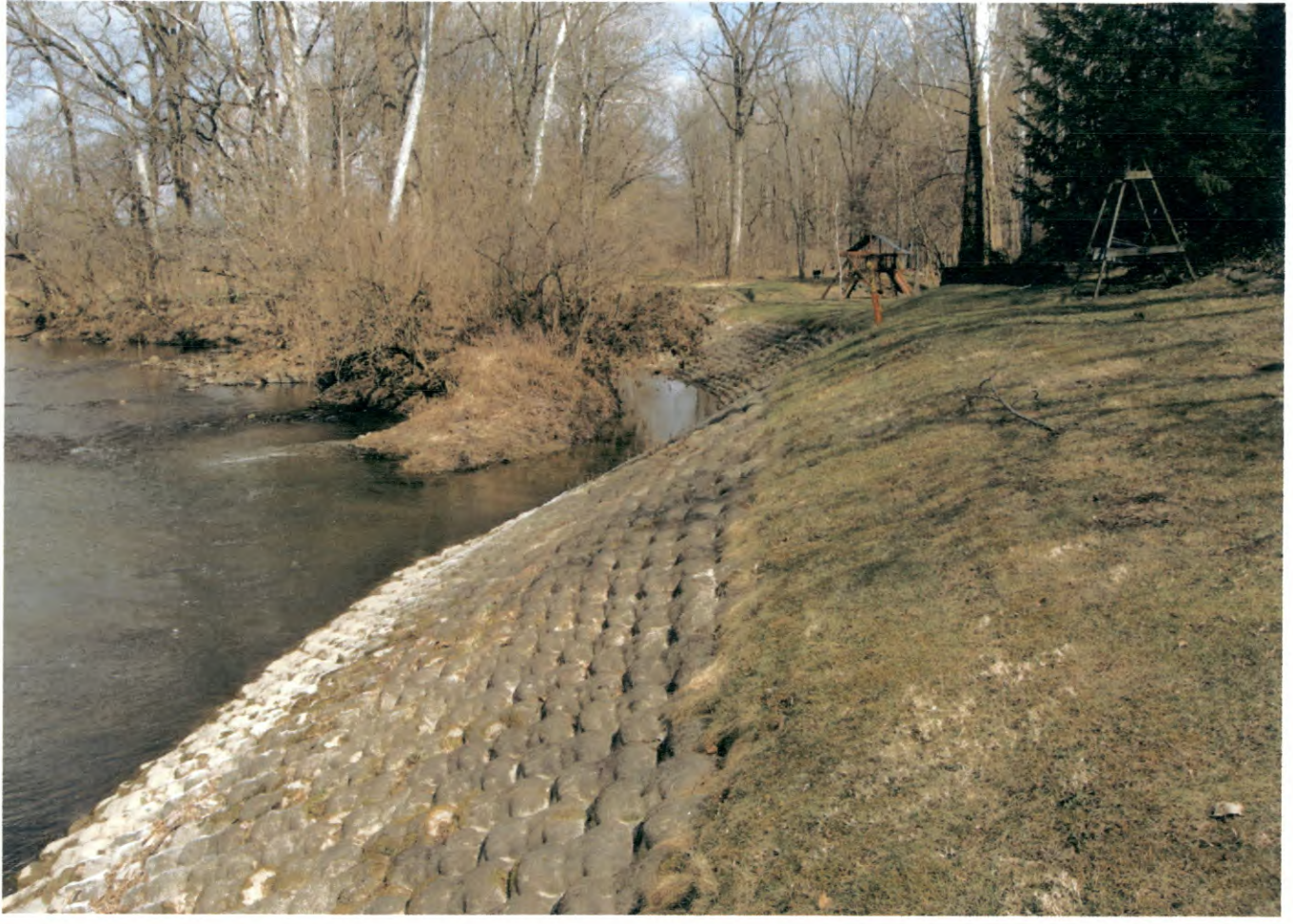
Little Eagle Creek North of 86th St. Fabric with Concrete. Looking North
