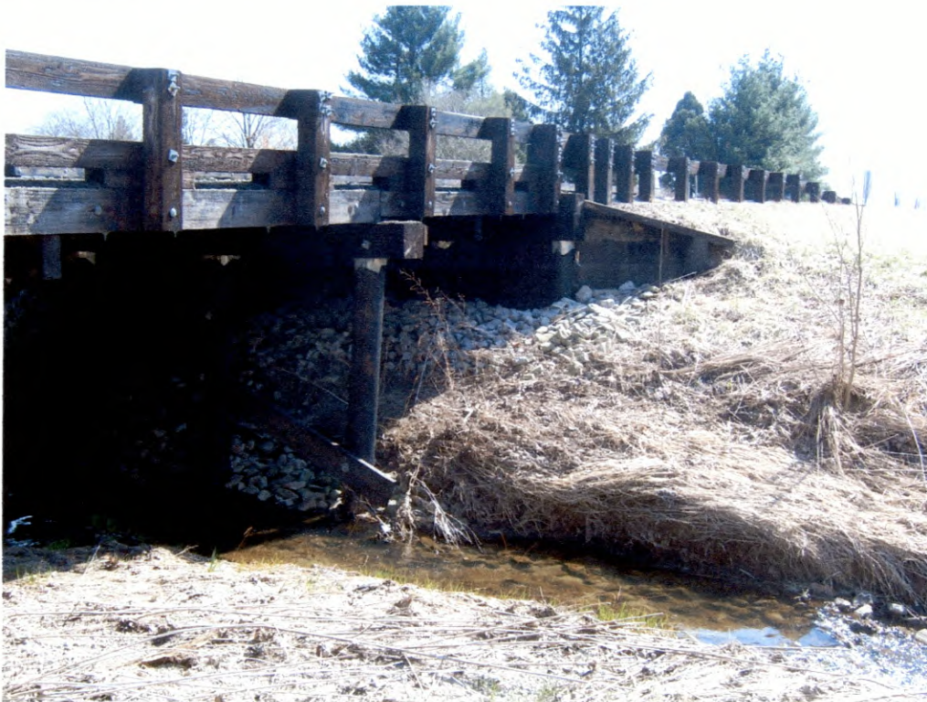
Picture of bridge south on Joliet Rd with minimal riprap and erosion control mats. Much better alternative, and has held up.
