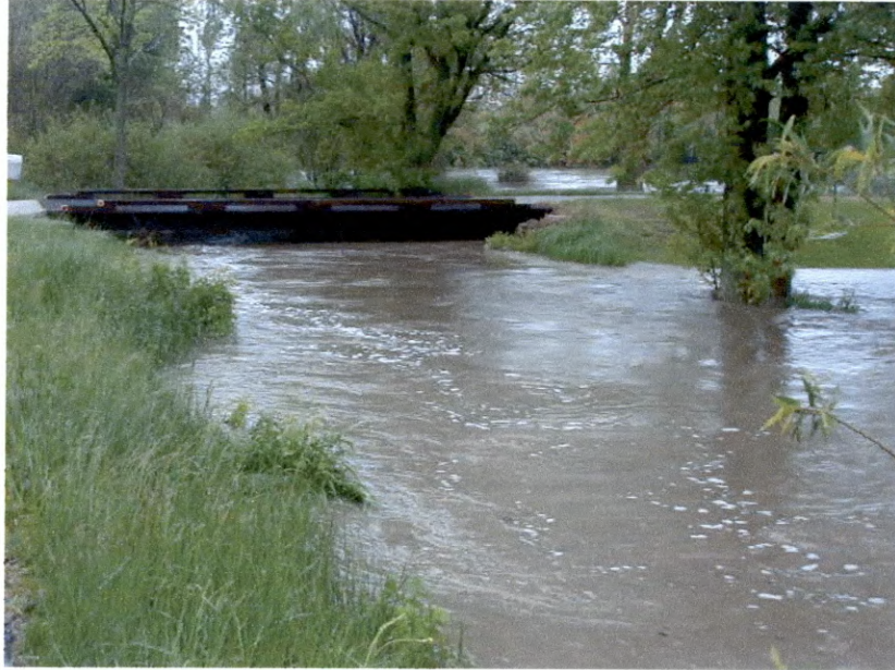
May, 2002. View from the road facing our bridge. Note the mailbox in upper left corner next to the bridge to get orientation for the next picture.
