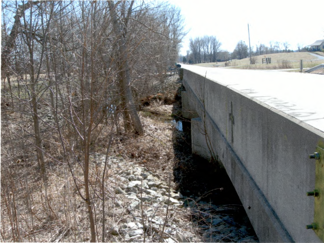
Picture of riprap north of my home on Johnson Gardner drain.
