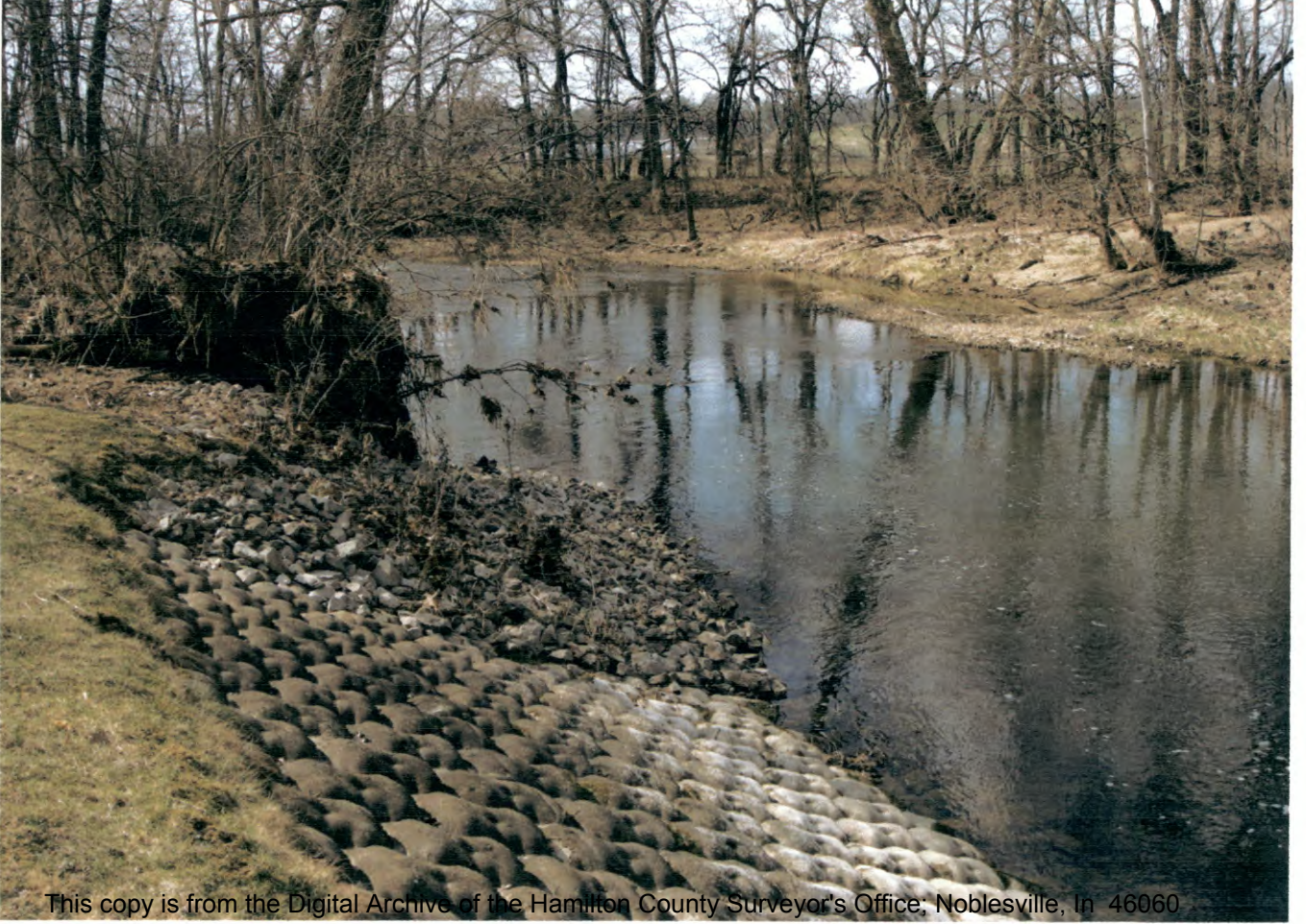
Little Eagle Creek North of 86th St. Looking South - transition to riprap
